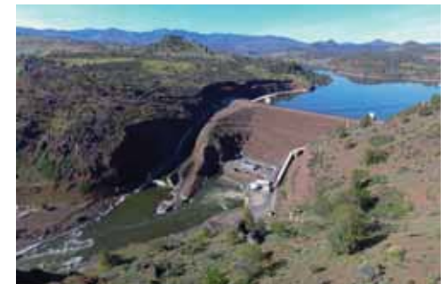
Iron Gate Dam. Photo: Mike Wier.
